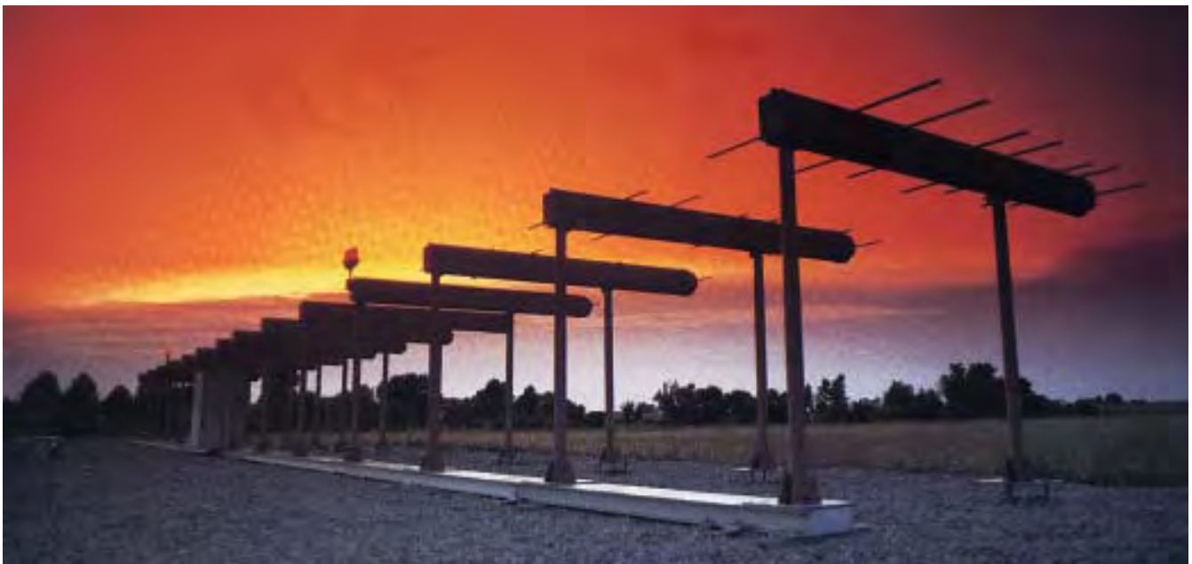
An array of antennas launches the localizer signal near the end of an ILS runway. The beams are beamed toward an airport runway at the right and reach out to about 50 miles.
